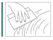
2• Apply an MS Polymer glue (eg Presto PM) to the underfloor using a 4x4 B3 trowel. Apply glue with "sweeping" actions in small areas, and never to the bottom surfaces of strips. You should use about 1.2 kg of glue per square metre.
